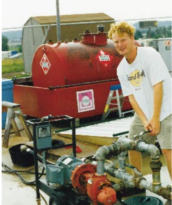
Jeff Wilcox, setting up to do a fuel transfer between tanks
