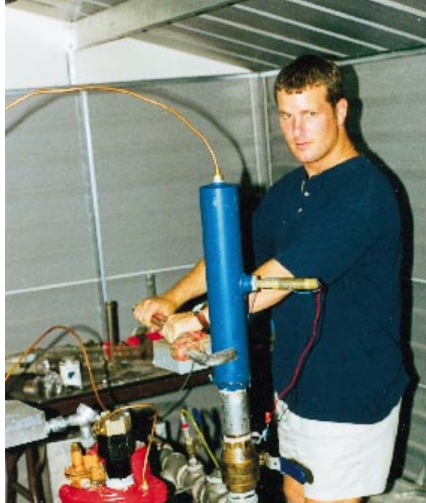
Craig Wilcox, installing a leak detector in a pipeline
